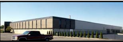
Overhead Door West Chester, Ohio Sold to First Industrial 90,000 SF
