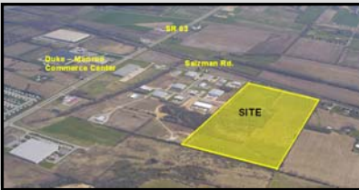
Monroe Logistics Center West Chester, Ohio Sold to IDI 80 acre industrial park
